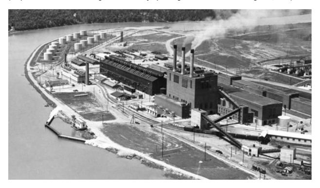
The S-50 liquid thermal diffusion plant for enriching uranium (the dark long building to the left of the Steam Plant) used steam heat from the world's largest steam powerhouse that was built to provide electricity to the nearby K-25 enrichment plant in case the power supplied by Norris Dam was interrupted.
